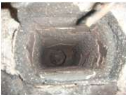
Fig-13 Bolt Area (Before Cleaning)
